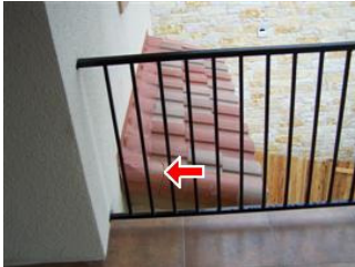
Damaged barrel tile
