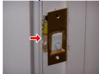
Light switch excessively gapped
